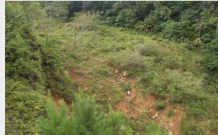
Figure 1: Current photo of an area where slippage has occurred
