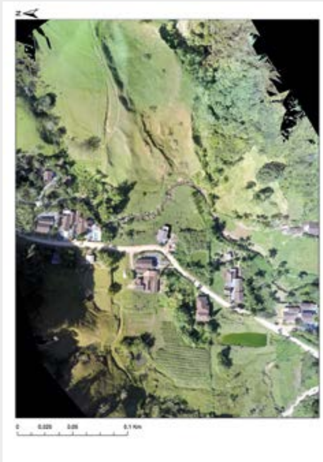
Figure 3: Photo generated from drone photo record
